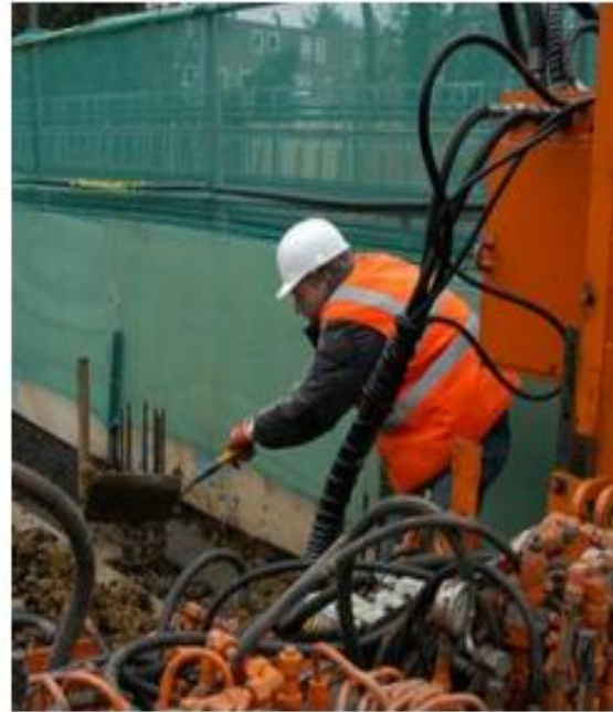
"construction worker in orange safety vest is working on road."
